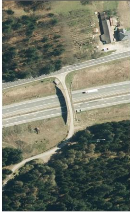
Overpass for wildlife at Les Tailles
