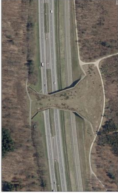
Overpass for wildlife at Grunhaut
