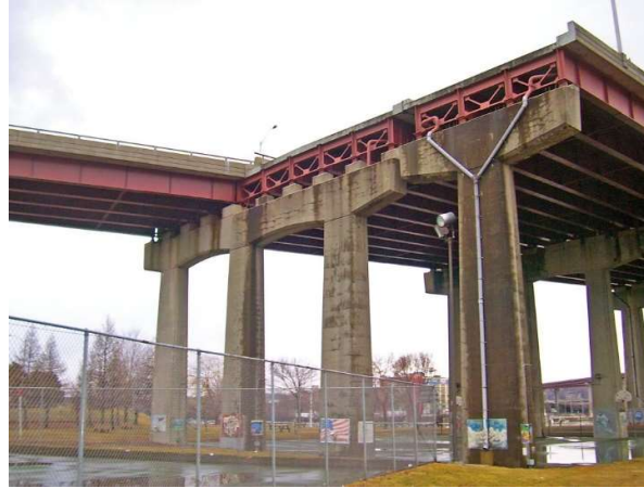
Figure 2 Deep cap beams in Dunn Memorial Bridge stub end (Wikipedia)
