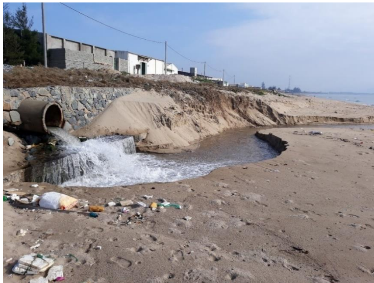
Figure 4 – Wastewater discharge in Ninh Thuan province
