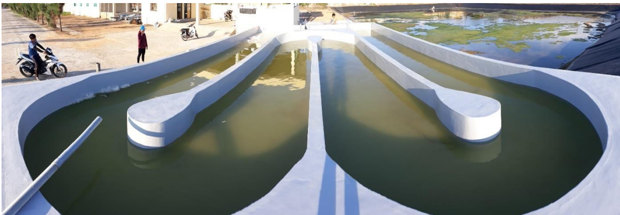
Figure 44 – HRAP pilot installed in the Ninh Thuan province
