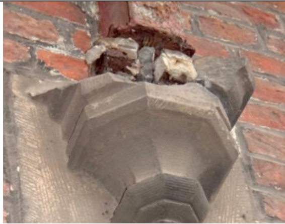
Figure 52: Corbeaux fracturé
