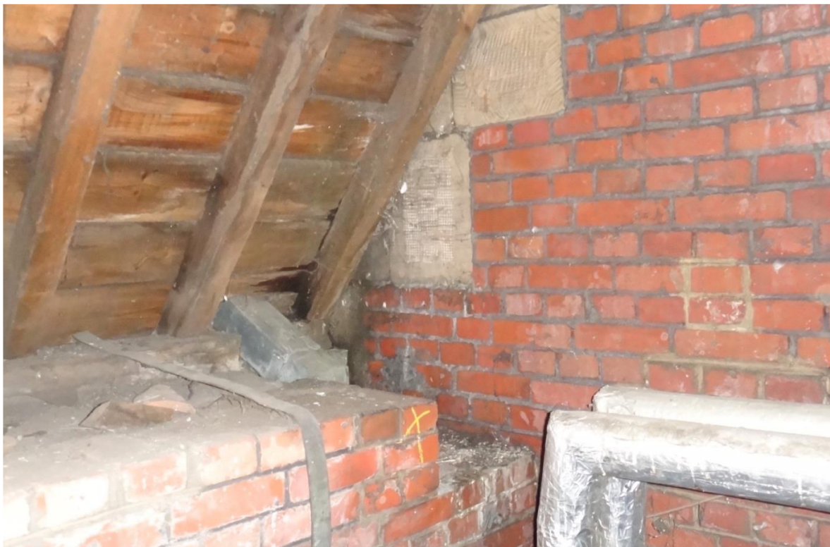
Figure 40: Photo de la charpente
