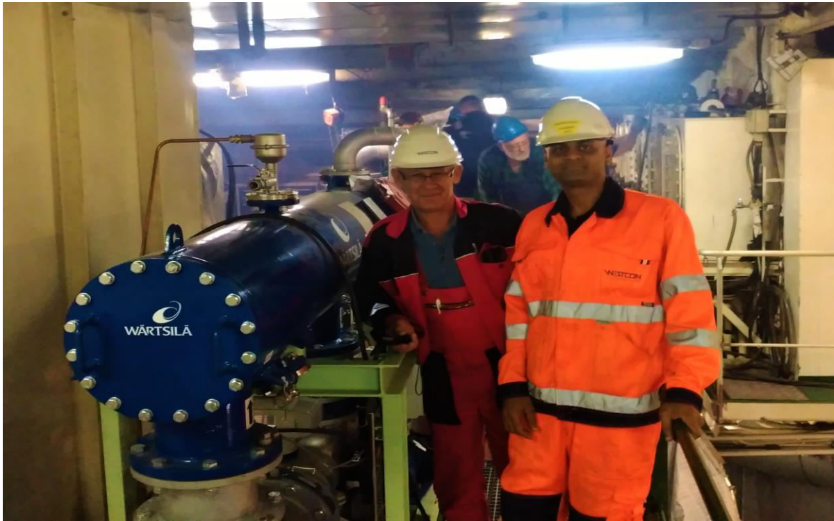
Figure 61: Inspection of installation by Mr. Andrzej Sobieraj (Internship supervisor) and author
