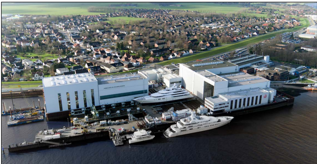
Figure 2: Air Photo of A&R Shipyard.
