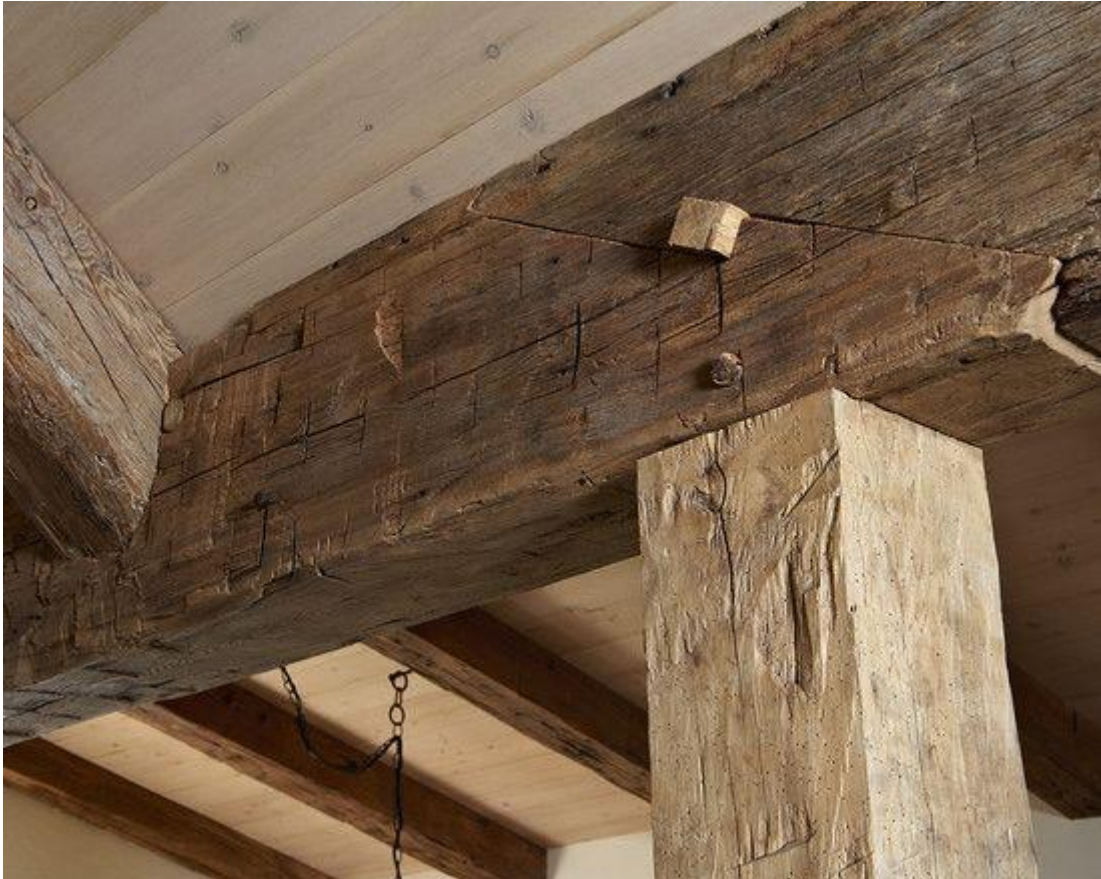
Figure 39 – Early example of scarf joint – roof construction
