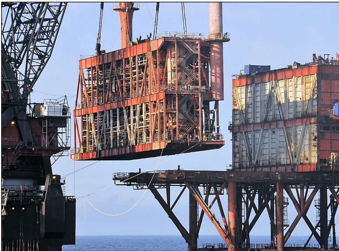
Figure 2 Example to removal operations
