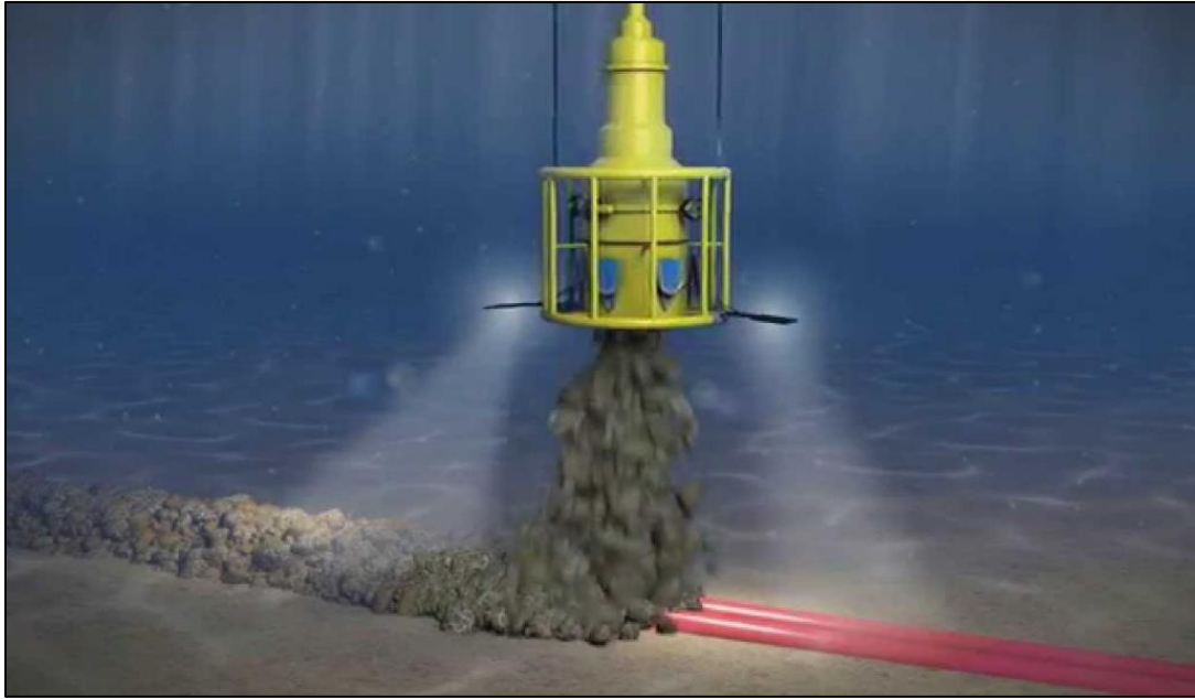
Figure 36 Application of rock dumping
