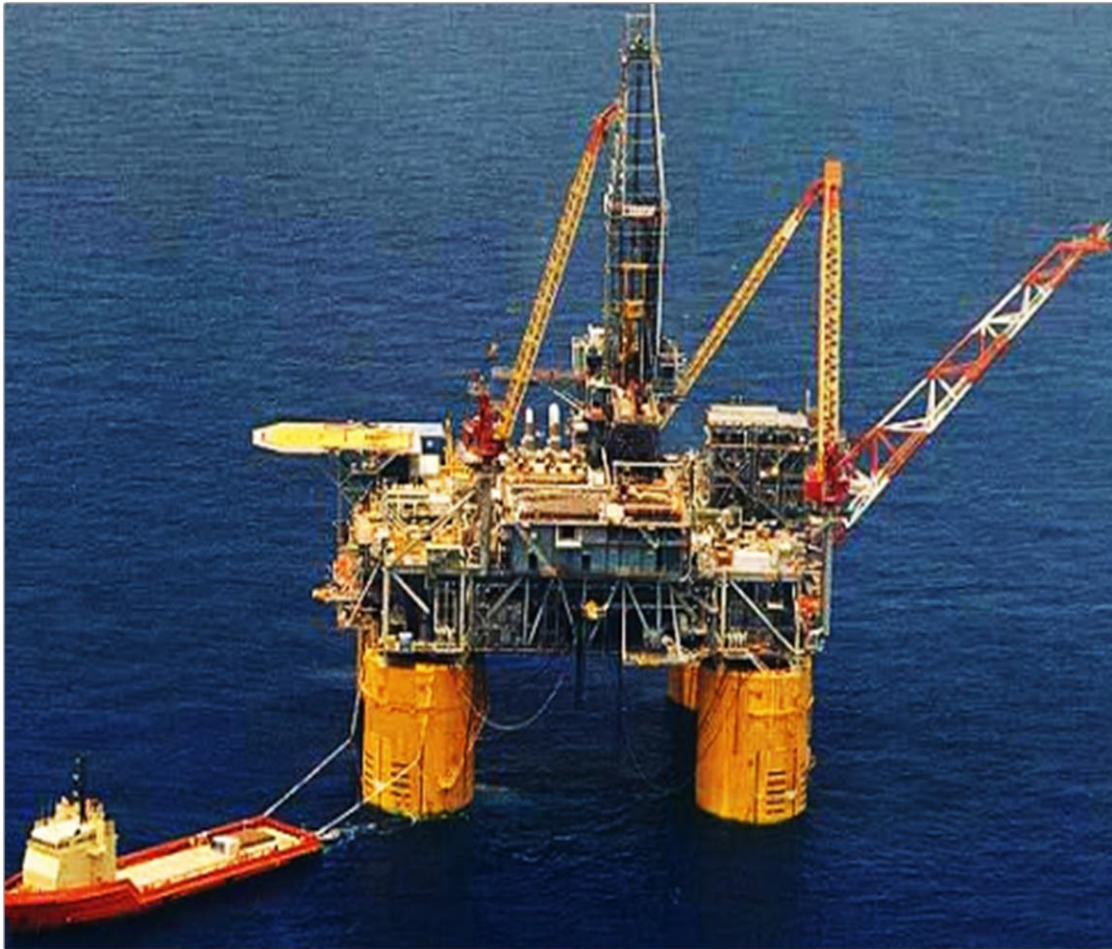
Figure 1 Typical offshore platform.
