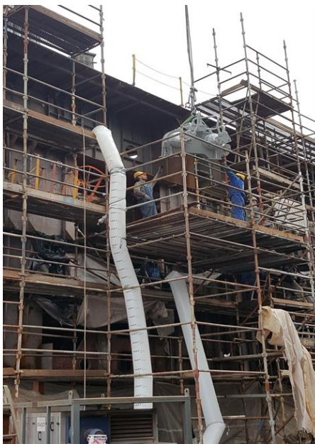
Figure 49. Fitters are introducing a dynamic pull component on-block. A good quality scaffolding system allows them to perform lifting maneuvers with safety and comfort. (source: fieldwork during internship at CRIST shipyard).
