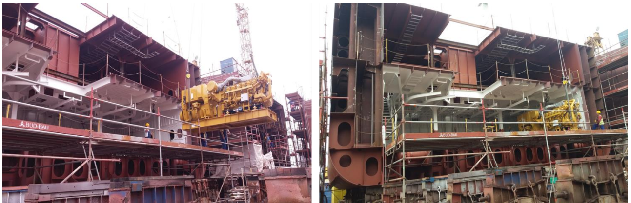
Figure 18. On-block advanced outfitting. Installation of a gen-set. (source: fieldwork during internship at CRIST shipyard)
