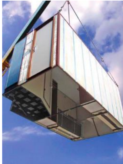
Figure 37. Installation of pre-fabricated cabin unit. (Source: http://img.nauticexpo.com )
