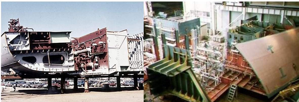
Figure 8. On-block outfitting sample. Pipelines. (source: http://i2.wp.com/lou.chirillo.com/wp-content/uploads/2014/06/AVON02k.jpg )
