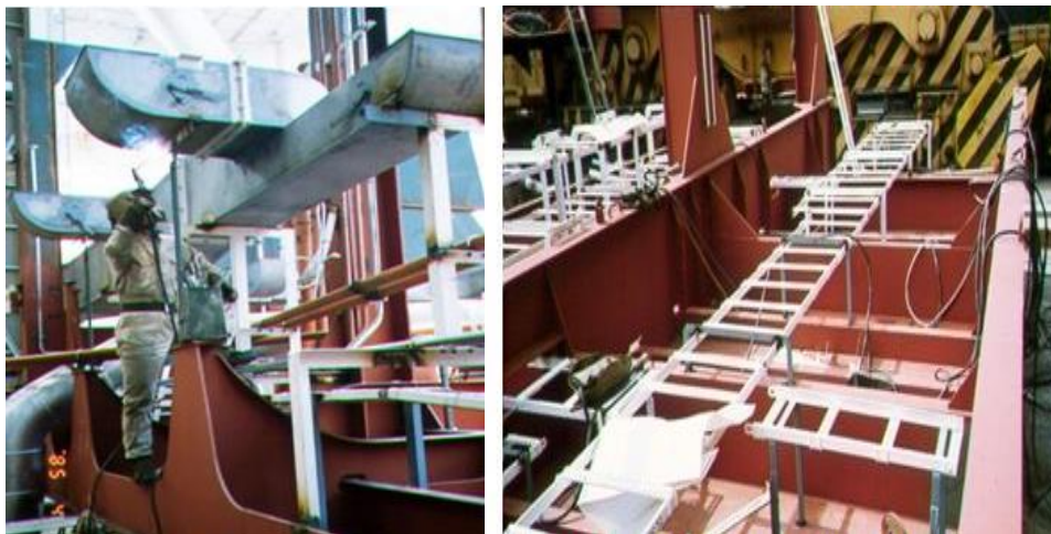
Figure 10. On-block outfitting sample. HVAC ducts installation and cable trays. (source: http://kalyan-sg.byethost22.com/MPM-II/On-Block-Example-01.jpg )
