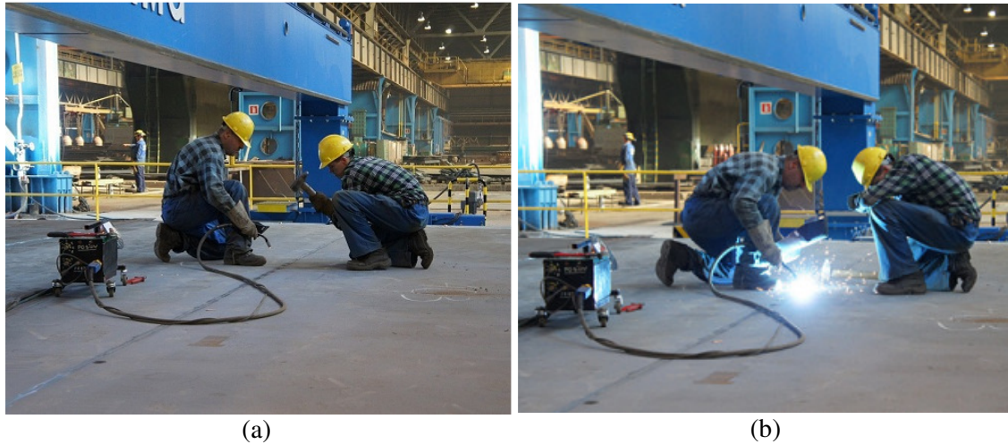
Figure 3.10 - Tack welding operation.
