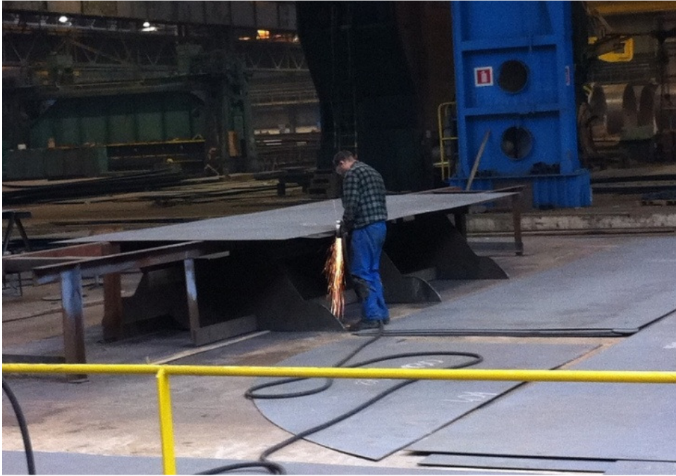
Figure 3.7 - Worker acting on edge preparation using pneumatic countersink.
