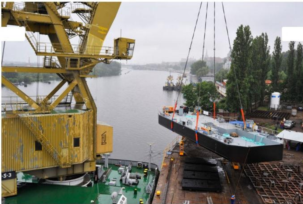
Fig.8.Ship launching by crane [14]
