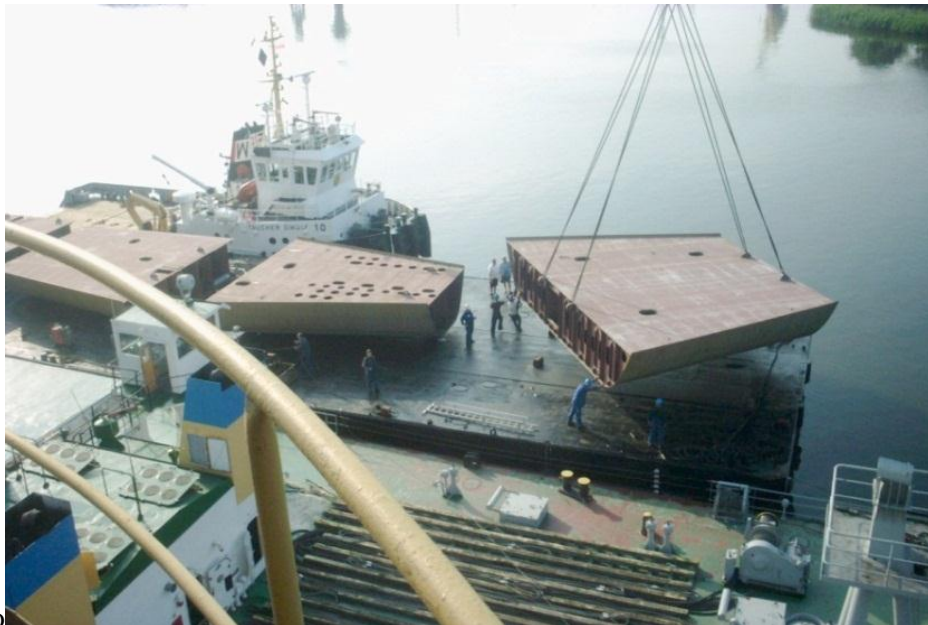
Fig.12.Transport of block by pontoon [14]
