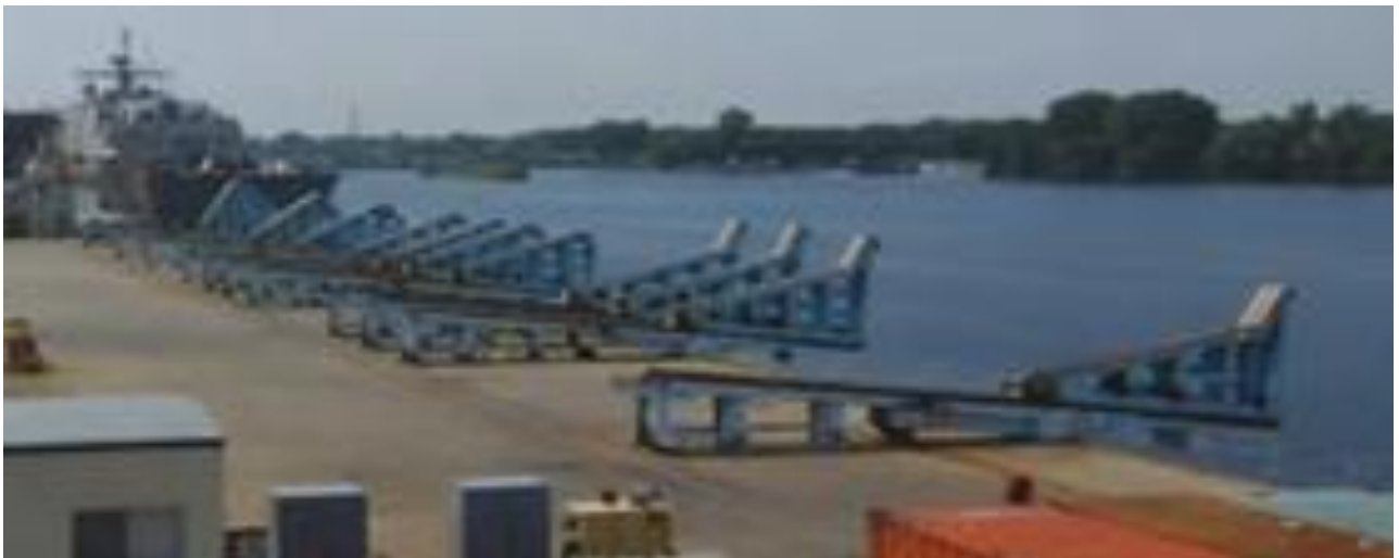
Fig.43.Slipway with different slip tracks [26]
