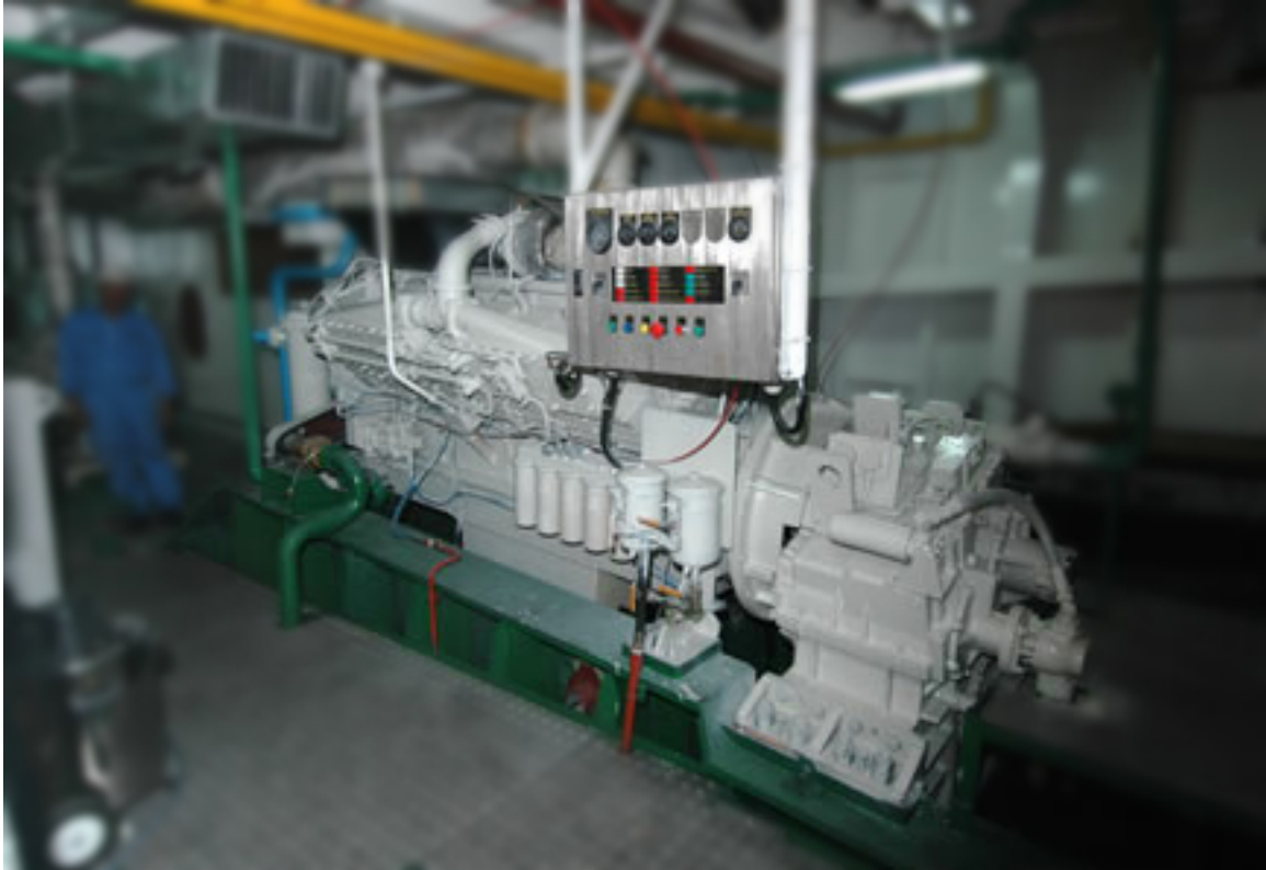
Fig.4.5 Sample engine foundation
