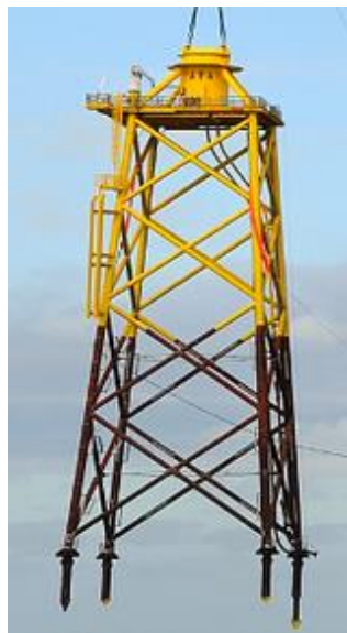
Figure 13: Jacket with jacket stab-ins. The right aft stab-in is longer and will be placed first in a pre-driven pile as a pivot. Picture available on http://www.lorc.dk/offshore-wind/foundations/jackets .
