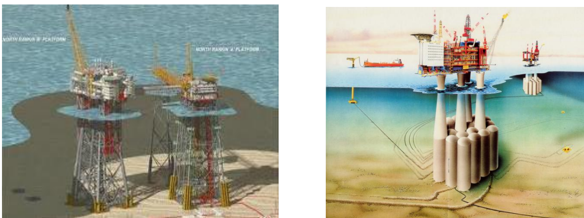
Figure 6 Jacket Fixed Platform (Left: Steel Jacket type Rankin Platforms, Source: www.project.connect.com.au ), Gravity-based structure (Right, Source: Prof: Tadeusz Graczyk Lectures at ZUT)
