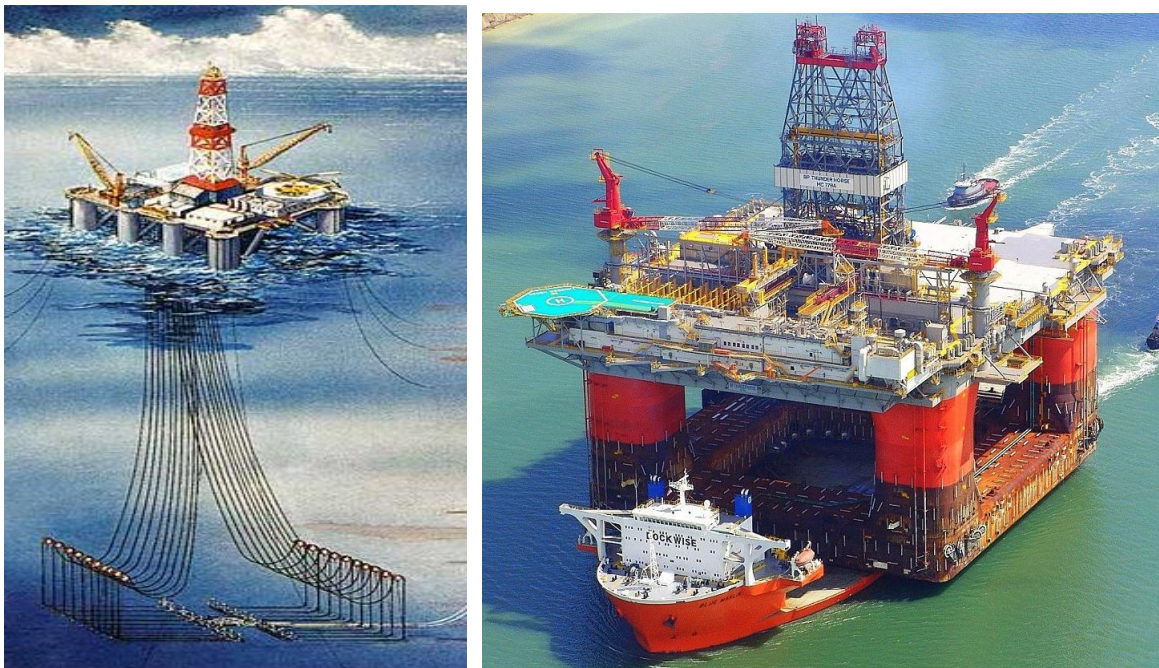
Figure 13 Left: Spread Mooring System of platform (Source: Offshore Technology), Right: One of the modes of Semisubmersible Platform Transportation, (Source: Dockwise)
