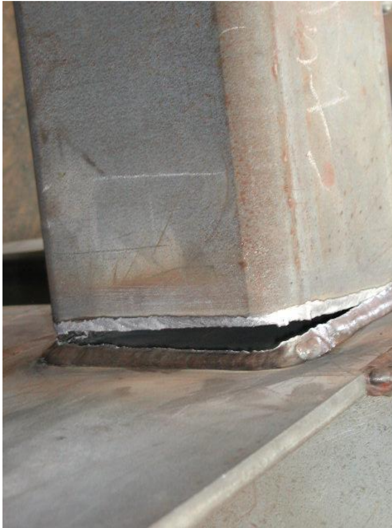
Figure 54: Pillar with 2 oblique reinforcement after breaking: 97.5 KN apply load © STX France
