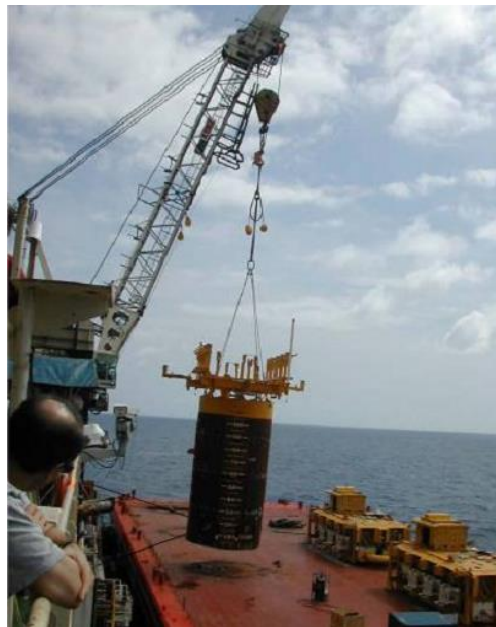
Figure 1- 1 Lifting suction anchor off transportation barge deck [1]
