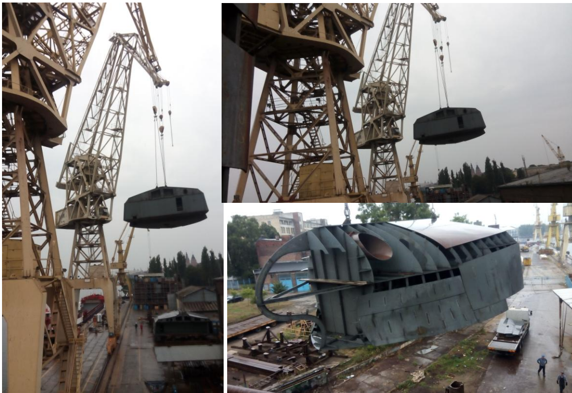
Figure 3.55 Transfer unit from fabrication shop to erection area
