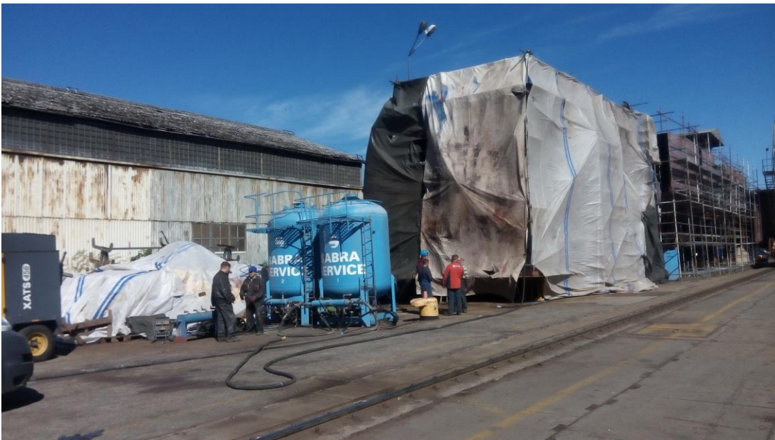
Figure 3.71 Surrounding plastic fence
