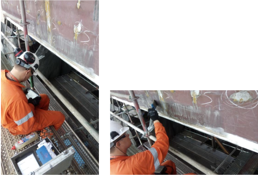
Figure 3.53 Radiography test on joint welding line in shell
