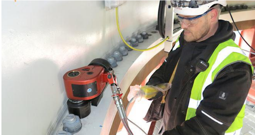
Figure 20: Pre-Stressing process (Kanbur 2014)
