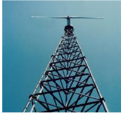
Figure 18: Lattice tower sample (“Everything You Need to Know About Small Wind Turbines” n.d.)
