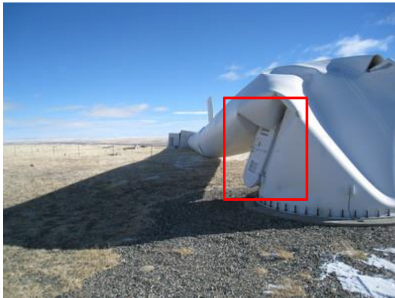
Figure 61: Wind tower accident due to wrong door opening estimation (“WindAction | Wind Turbines and Public Safety: Setbacks Matter” n.d.)
