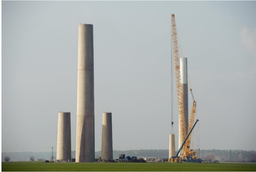
Figure 22: Concrete towers for wind turbines (“ACCIONA Windpower Inaugurates the First Concrete Tower Production Plant in Mexico” n.d.)
