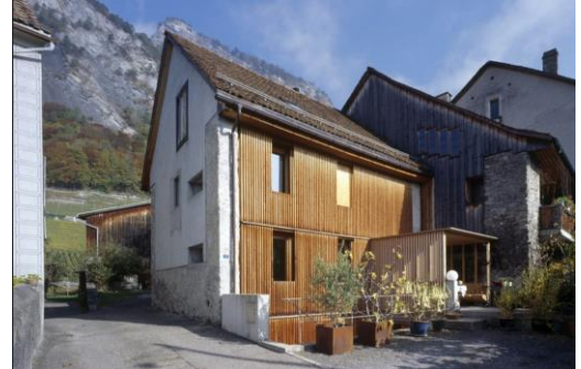
Figure 31 : photo G. Bally - Fläsch
