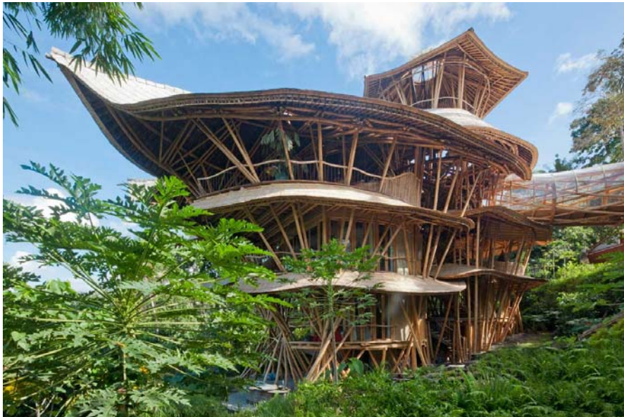
FIGURE 30 - SHARMA SPRINGS RESIDENCE, GREEN VILLAGE, BALI, BY IBUKU
