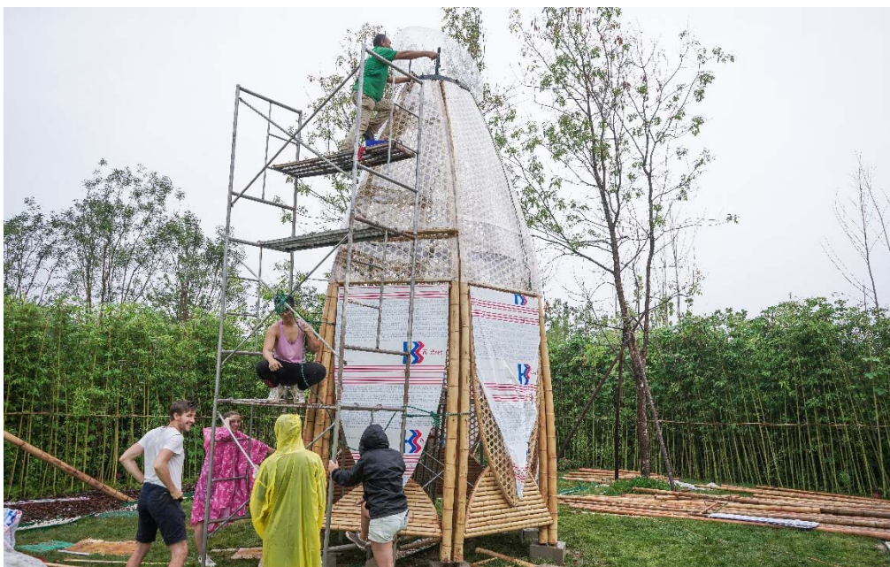
FIGURE 59 - MOUNTING THE HOUSE LOTI PAVILION ON-SITE, PERSONAL COLLECTION OF PHOTOGRAPHS
