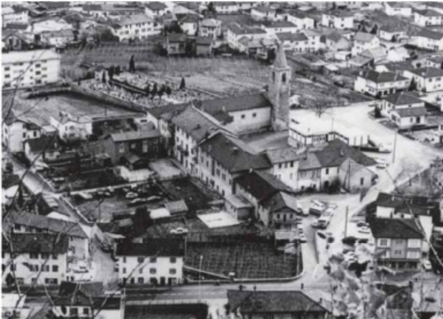
Figure 60 : Monte Carasso avant intervention
