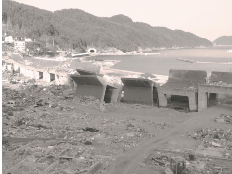
Figure 2 Partially Damaged Sea Wall (Iwate Prefecture: June 9, 2011) [1]
