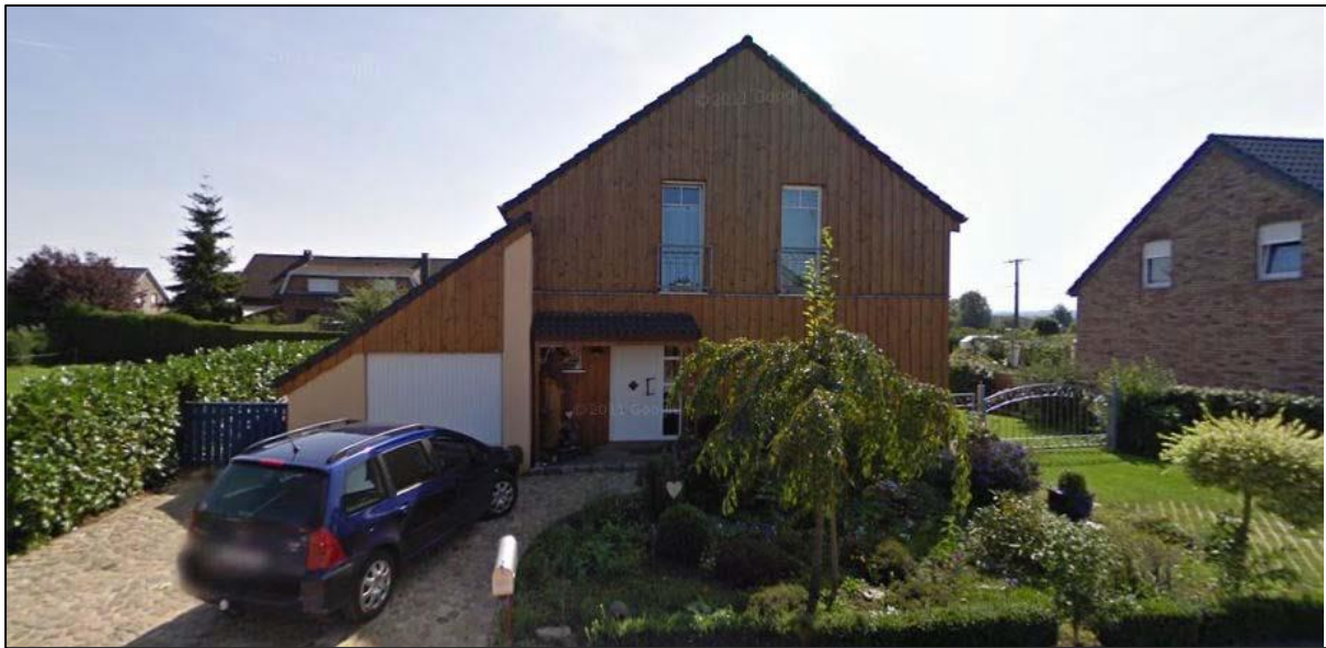
Figure 3.5-The Kettenis House. Source: De Meester,2008.
