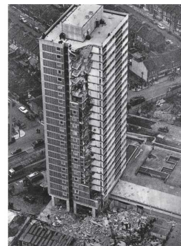
Figure 1.2: Ronan point collapse 2 .
