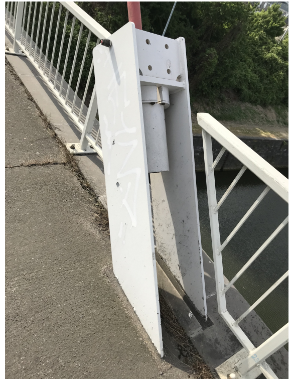
Figure 3.15: Picture of the connector and the anchored support.
