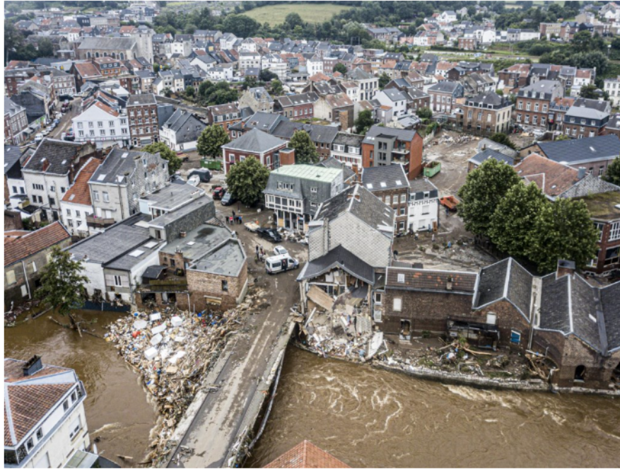
Figure 2.23: Real clogging of the bridge francval
