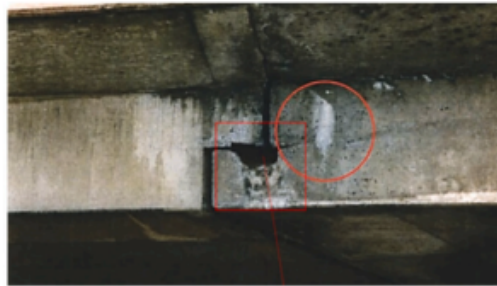
Figure 1.2: Deteriorated dapped-end connection [30]
