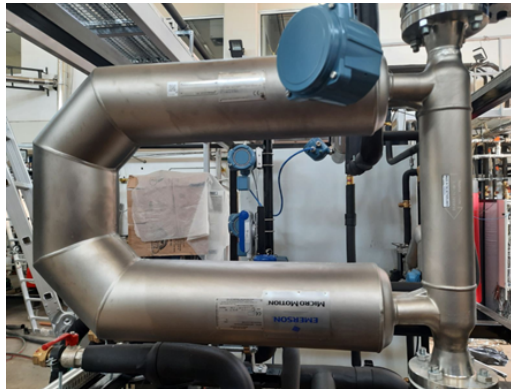
Figure 3.6: The installed CMF200 Coriolis flow and density meter of Emerson Micromotion Elite series.
