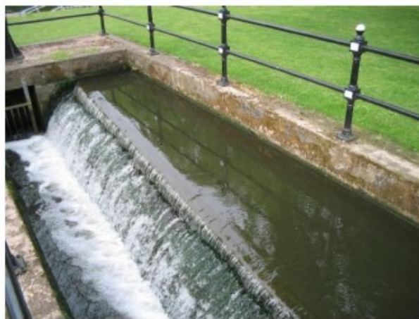
Figure 2.5: Flow over a side weir
