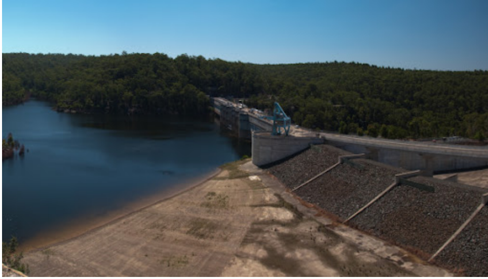
(a) Photo of earth fuse plugs at the Warragamba Dam in Australia (from Reid)
