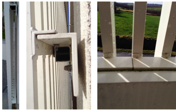
Figure C.1 – Real view on site of cylinders fixation
